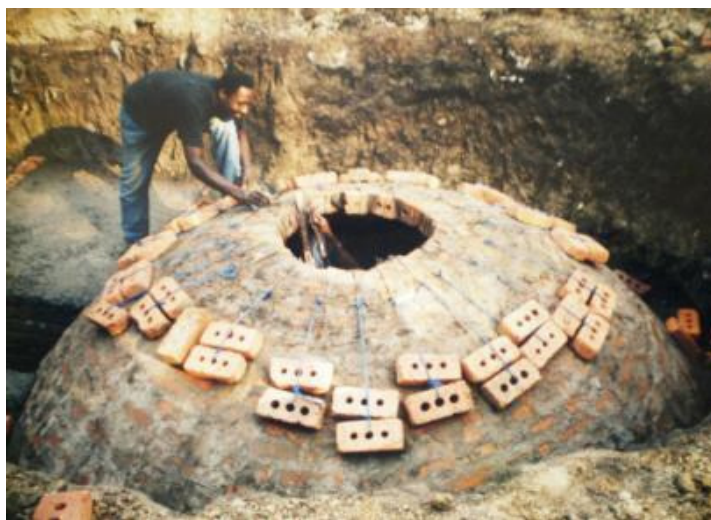
Construction of biogas facility in Ghana
