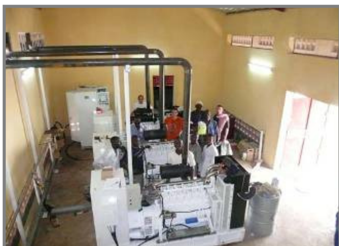
The three Garalo gensets in position (left). The power house at night producing power for the village (right).
