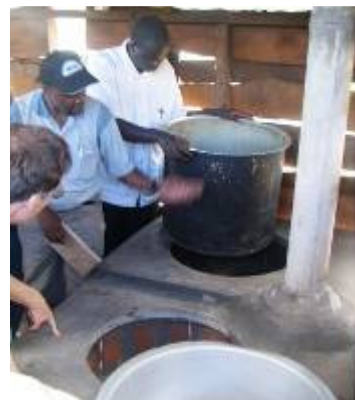
Improved cookstove installed at Noseiya Primary School in Leguruki.
