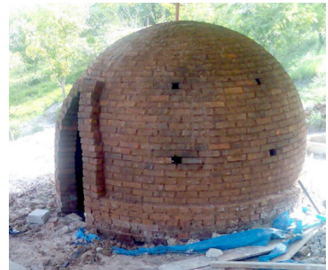
Half Organge Kiln for charcoal production
